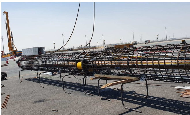
Photograph 1. BDSLT pile installation
