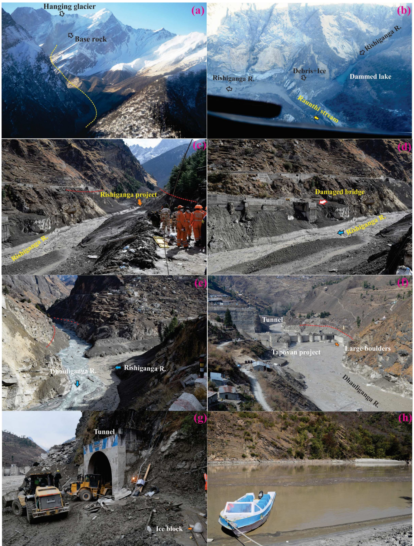
Fig. 2. View of the triggering site of the ice-rock avalanche (a), lake formation at the confluence of Raunthi stream with Rishiganga River (b), damaged site of Rishiganga HEP (c), washed out bridge near Raini village (d), signature of back thrusting at the confluence of Rishiganga and Dhauliganga rivers (e), deposition of slurry material at Tapovan HEP barrage (f), tunnel (g), and high SSC in downstream (h).
