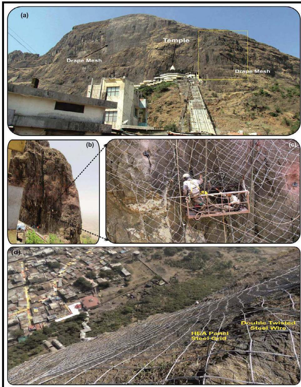
**Fig.10.** Proposed rockfall mitigation measures: **(a)** Implementations of drape mesh, **(b)** in-large part of yellow rectangle in **a**, **(c)** workers installing drape mesh along with rockbolts, **(d)** installed double twisted steel wire and HEA panel steel grid.
