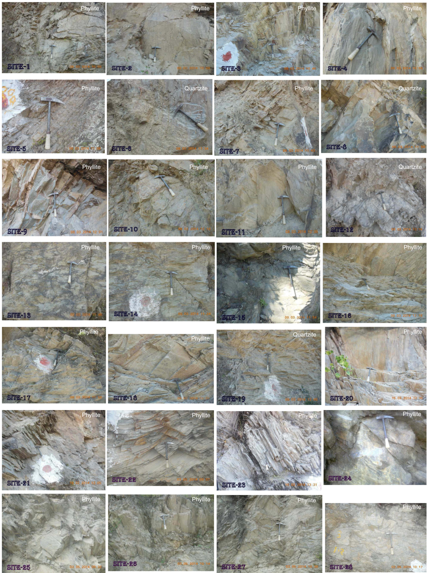
32 rock slopes/rock cum debris slopes identified in the study area
