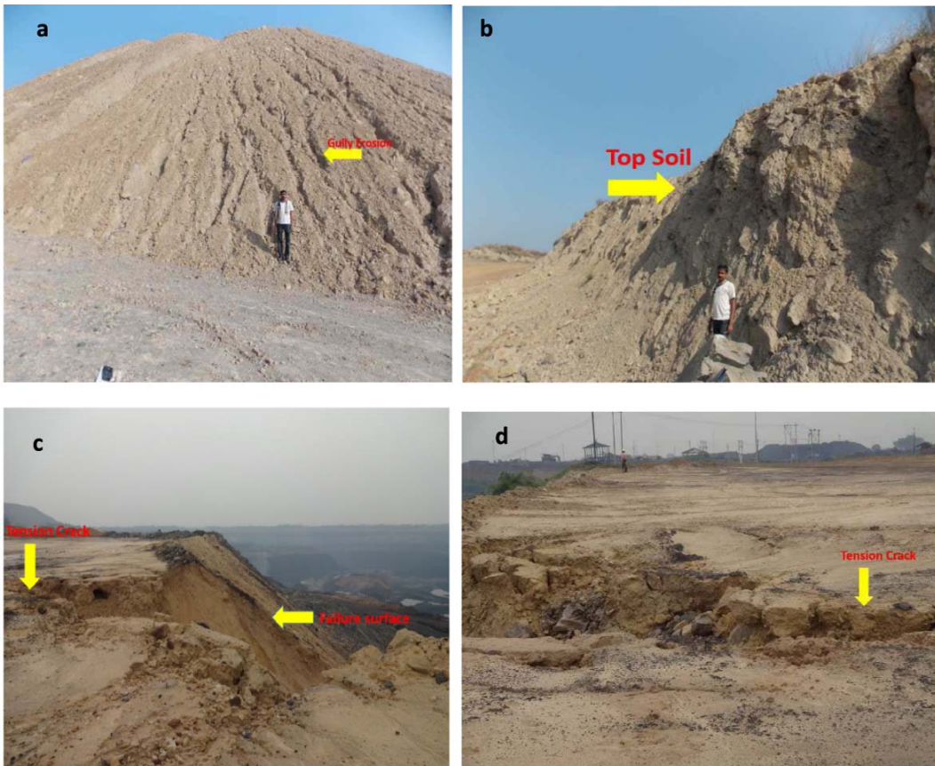
Fig.5. Field photographs showing: (a) Gully erosion, (b) Weathered top soil, (c) Failed dump slope, (d) Tension cracks.
