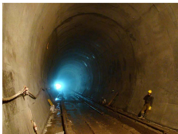
Fig.7. The rounded shape of the tunnel (after final lining)
