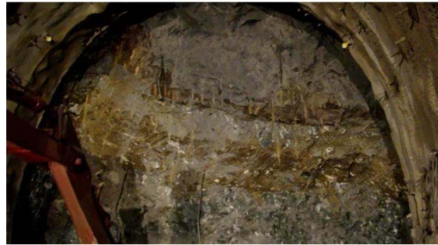
Fig.5. Fault gouge demarcating the conglomerate of the Siwalik Group in the upper portion and the mudstone of the Murree Group in the lower portion
