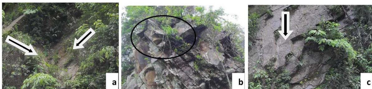
Fig.7. (a) Wedge failure. (b) Toppling failure and (c) Planar failure
