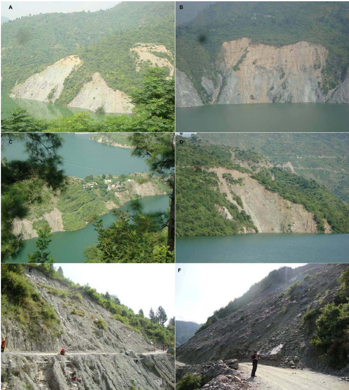
Fig.9. A,B,C and D refers to the landslide incidences along the side slopes adjoining the reservoir where as E and F shows the landslides incidences on the steep cut slopes along the road.
