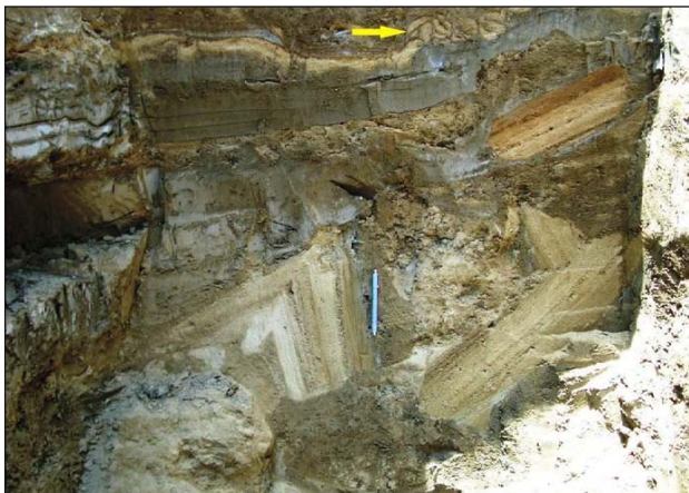
Fig.5. Photograph of the northern wall of trench-2 showing collapsed blocks of hard cap sediments. The blocks also contain coarse to fine sands that ejected during the earlier episodes of liquefaction. Note the complex mixture of liquefaction sands and clays with minor convoluted (mentioned by an arrow) beds indicates reactivation of the vent many times during several aftershocks.
