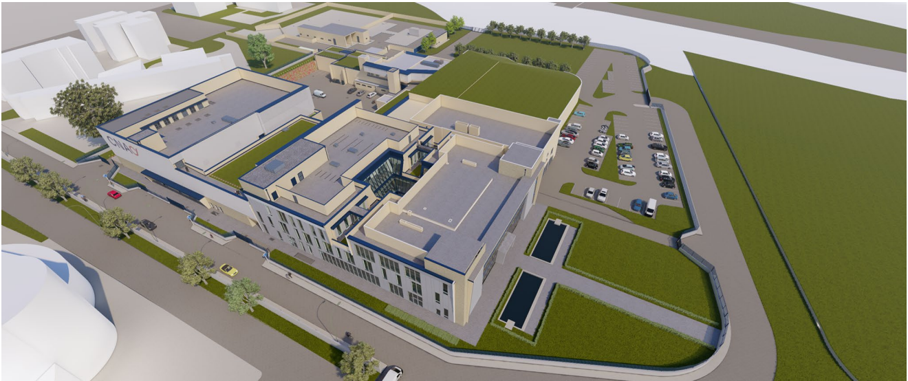
Fig. 5 Render of the CNAO facility after the completion of the expansion works
