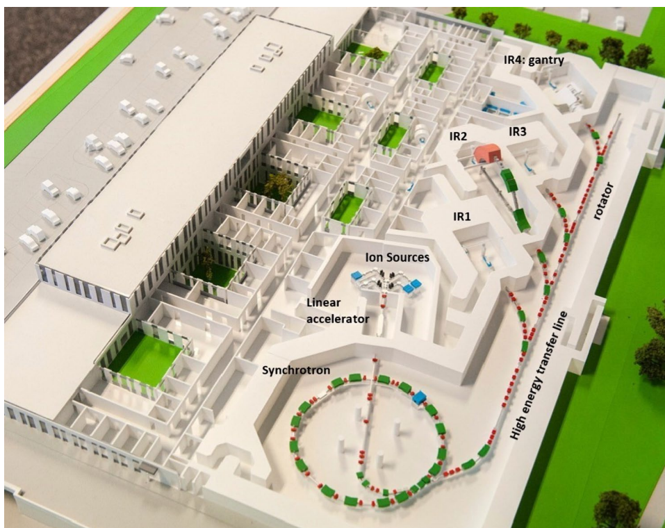
Fig. 4 Bird view of the MedAustron facility representation including the ion sources, the LINAC first stage of acceleration, the synchrotron, the extraction to the HEBT and the rotator and the four irradiation rooms including the gantry
