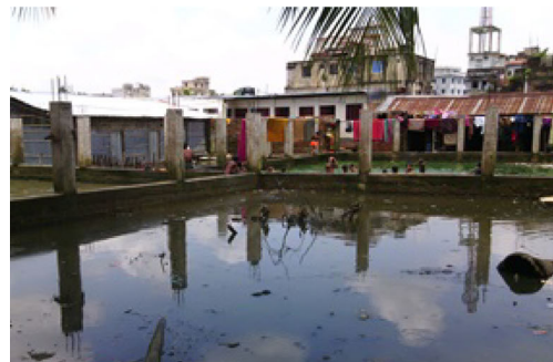
Concrete fills on pond for building new homes in Bakolia area
