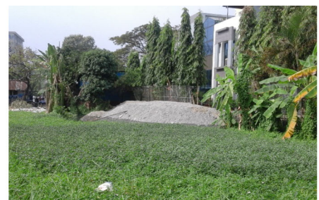
Pond filled-up for expansion of land in Muhammadpur area south Shaloshar
