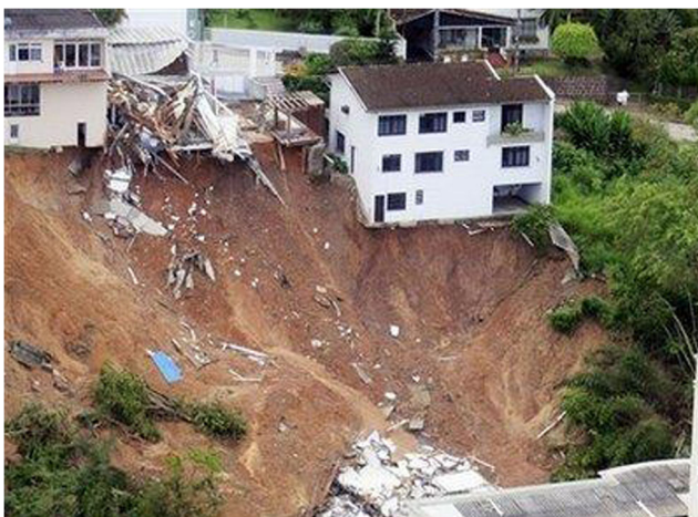
Fig. 2 An example of damage caused by landslide (Brazil)
