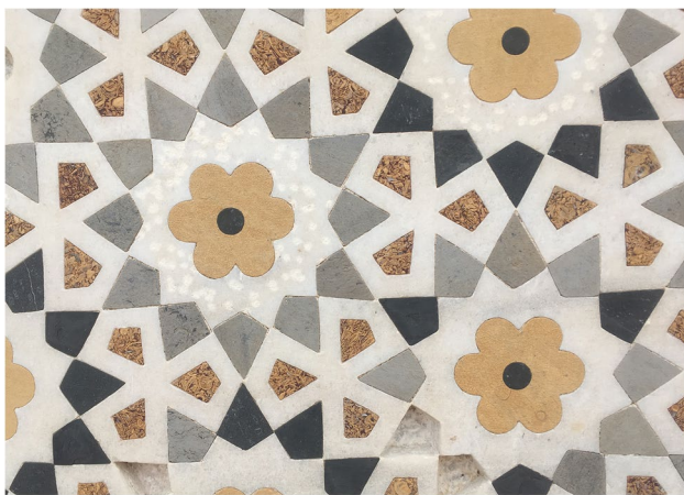
Fig. 5 Close-up of a panel on the exteriors. The pattern indicates that the grey and black coloured stones were ostensibly of the same (black) colour when originally fitted in place
