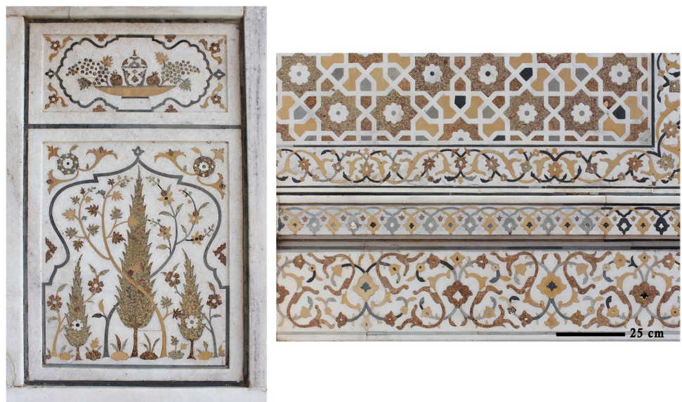
Fig. 2 Details of the inlay work on the exterior of the tomb showing intricate motifs and patterns attained by embedding different coloured stones in a white marble base
