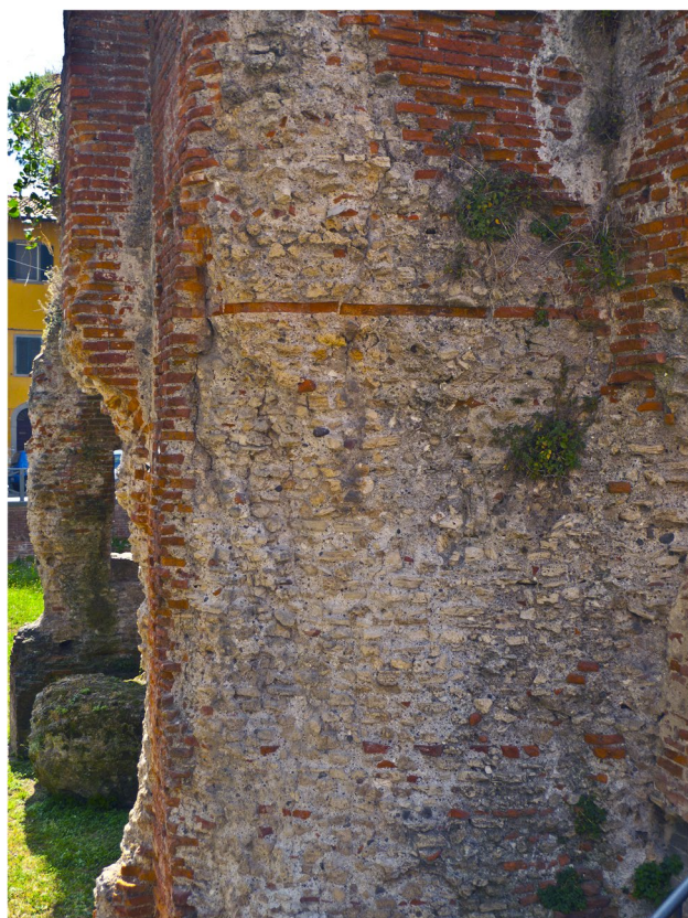
Fig. 9 A typical Roman brick-faced concrete wall with bipedalis bonding courses. Broken bricks and stones are used as caementa and are layered in horizontal courses, to achieve maximum strength of masonry (Baths of Nero, Pisa, Italy)
