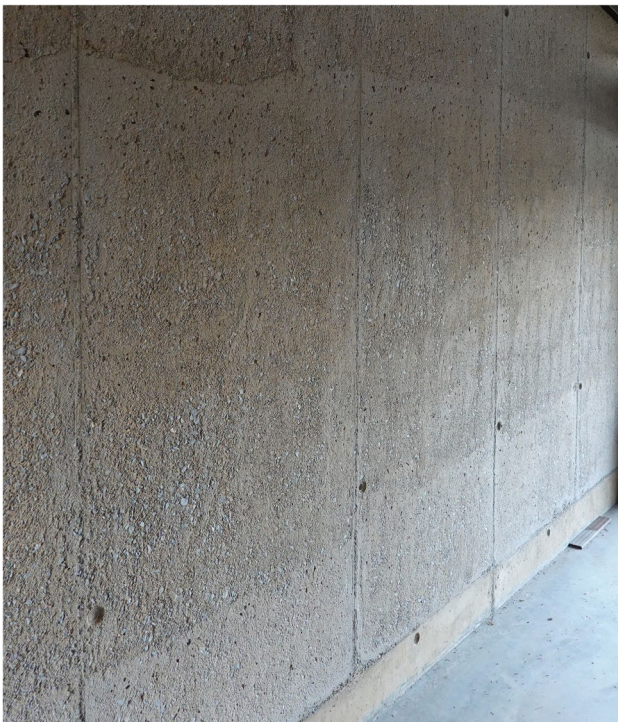
Fig. 1 Modern concrete wall (Cruilles, Catalonia). The undulating layers of concrete derive from the pouring process. One- to 3-cm size aggregates are entirely bonded by the Portland cement paste
