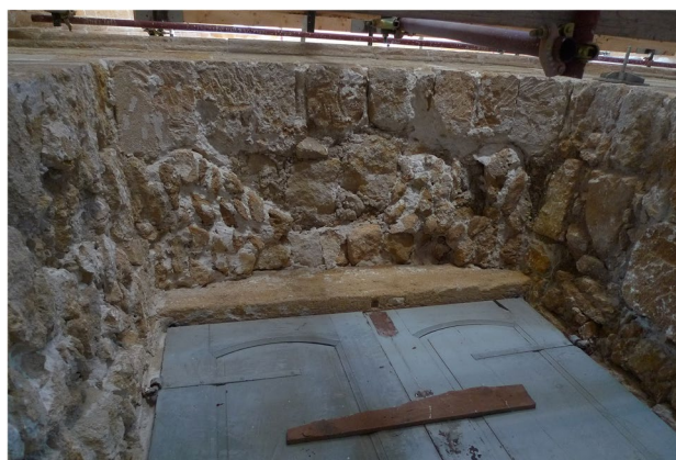
Fig. 16 Gypsum mortared rubble masonry at the Armenian Church at Nicosia, Cyprus
