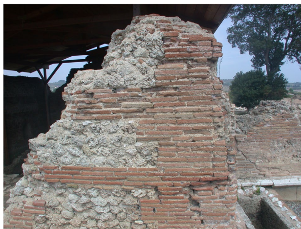
Fig. 10 Brick horizontal bonding courses in a rubble masonry wall (Nicopolis, Greece)
