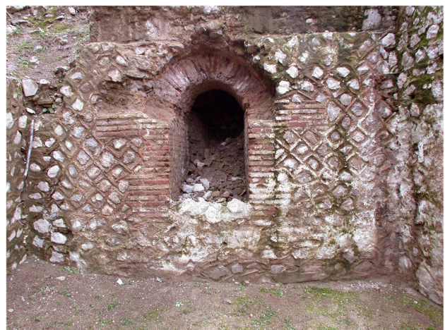
Fig. 8 Stone-brick reticulate in the stadium of Patras (Greece). Bricks are used to reinforce the bond between the facing and the core
