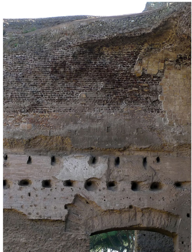
Fig. 14 Roman concrete barrel vault. Caementa made from red volcanic scoria layered horizontally (Baths of Caracalla, Rome, Italy)
