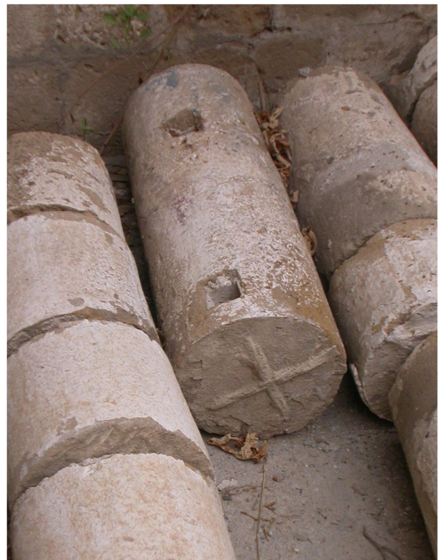
Fig. 12 Drums of a column in the Armenian Church of Nicosia (Cyprus) showing the imprint left on the mortar by cross-shaped groove made to increase the mortar joint of an otherwise thin joint. Other grooves have the shape of a trident
