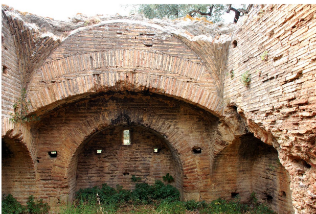
Fig. 15 Solid brick arches and vaults in a Roman tomb at Troezen (Greece)
