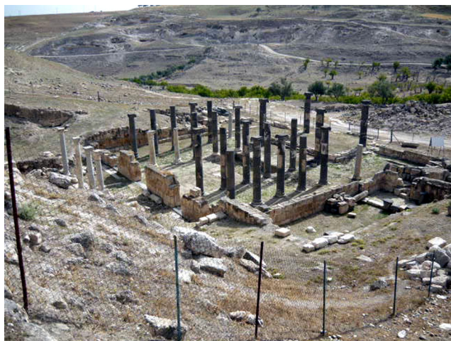
Fig. 4 The columns of the cruciform basilica (facing northeast)
