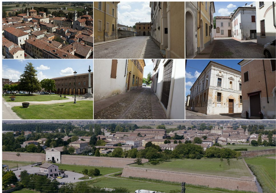
Fig. 1 Several photographs showing Sabbioneta, the historic city used as a case study in this article. The pictures show some of the town's streets, characterized by various widths, and buildings leaning against the street; the fortified walls and a square can also be seen
