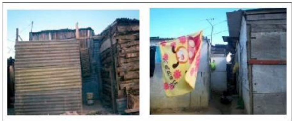
Fig. 13 Informal housing units (shacks), the structures generally have heterogeneous roofing materials
