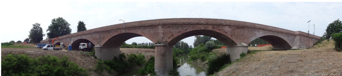
Fig. 2 The test site: “Motta di Cavezzo” bridge (Modena, Italy)
