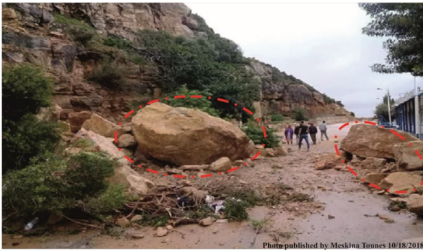
Fig. 1 Big rockfall blocked the road to Korbous
