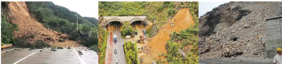
Fig. 1 Landslide hazards at tunnel entrance section
