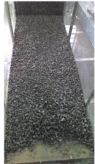
Fig. 5 Laying of drainage layer (gravel layer)
