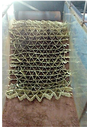
Fig. 16 Placing of bamboo geocell over compacted 60° slope
