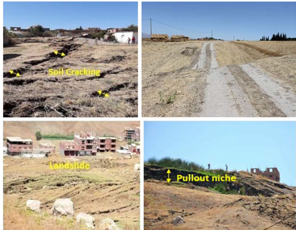
Fig. 4 Examples of the most recent landslides occurred in 2020 that caused ground deformations and severe damage to buildings, roadways, and public infrastructures in the urban area of Mila city (Bounemour 2019)
