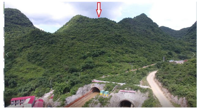
Fig. 2 Tunnel top of water gushing section
