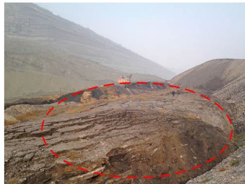
(c) the heave in the bottom of the slope
