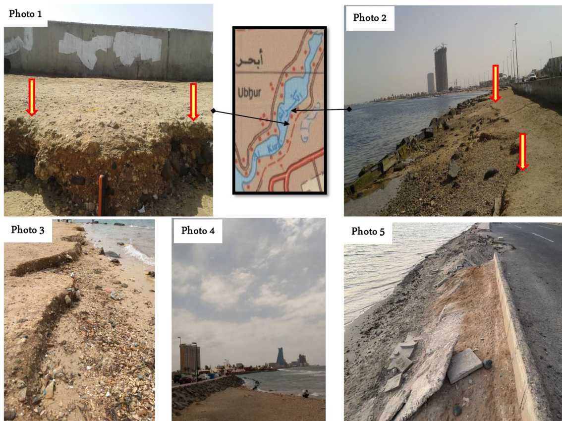
Fig. 9 Manifestations of erosion in northern part of the coast: photos 1 and 2 were taken in 2015, photos 3 and 5 in 2019, photo 4 shows some measures taken against erosion. Source: Authors
