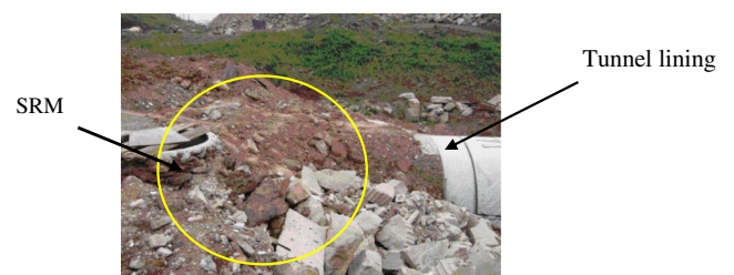
Fig. 3 Investigational area of SRM in tunnel site
