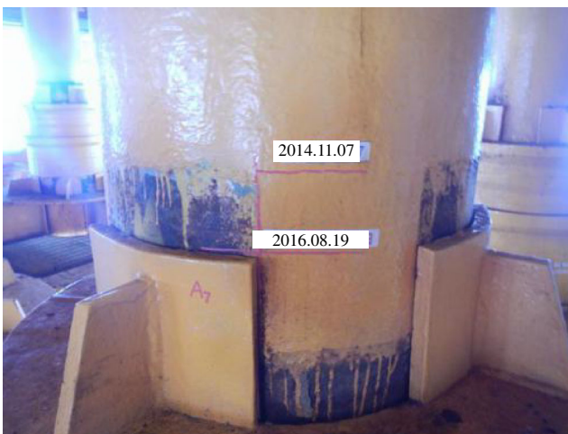
Fig. 2 Marine riser uplift
