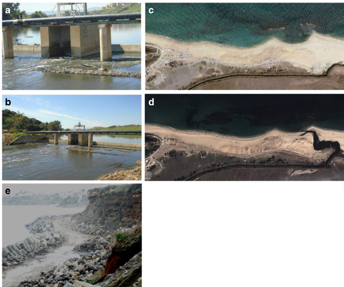
Fig. 9 a, b The valve of separation between the Reghaia River and the Reghaia lake (sediment trapping). c, d Deviation of the Reghaia mouth river. e Seawalls installation in Ain Taya
