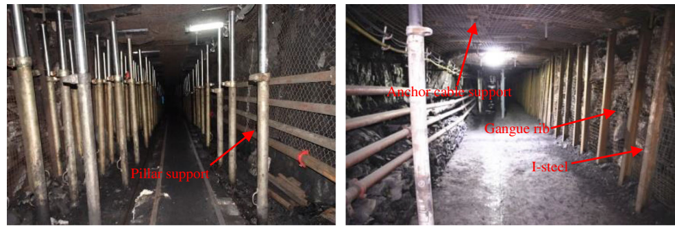
Fig. 18 The formed roadway in the 8501 working face
