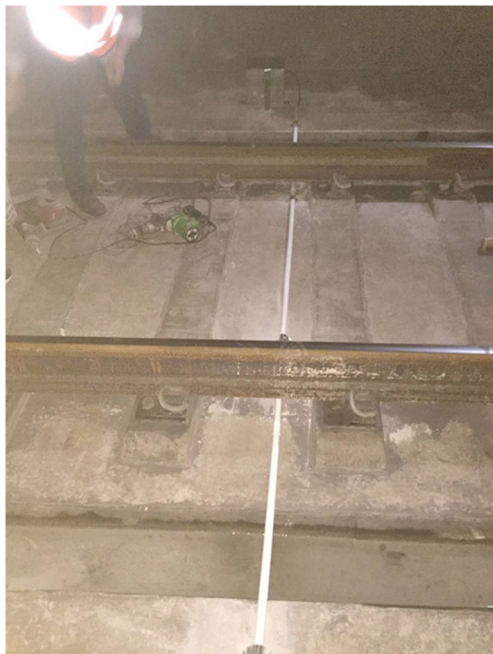
Fig. 12 Cable crossing
