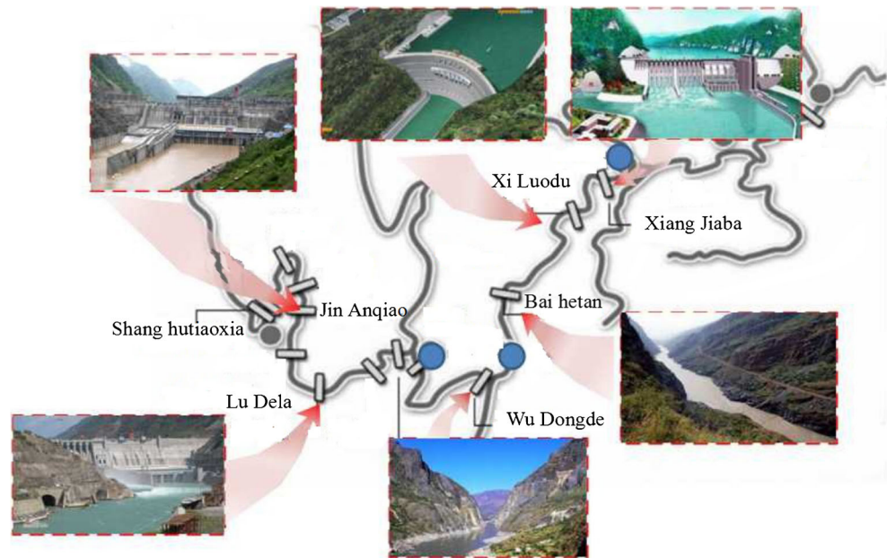
Fig. 13 Dam constructions on the upper Yangtze River
