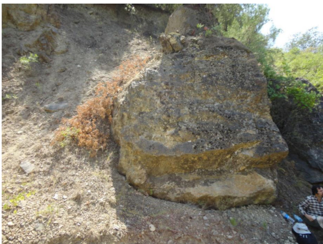
Fig. 6 Rock blocks removed by the mass movements
