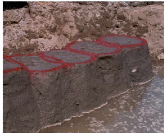
Fig. 2 i Illustration of the jet grouting procedure. ii Photograph of field implementation of jet grouting (source: http://www.chemicalgrout.co.jp/en/ ). iii Photograph of overlapped jet columns in sandy soil obtained from field trials (source: http://www.kftco.com/ )
