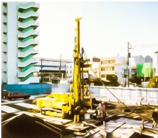
Fig. 2 i Illustration of the jet grouting procedure. ii Photograph of field implementation of jet grouting (source: http://www.chemicalgrout.co.jp/en/ ). iii Photograph of overlapped jet columns in sandy soil obtained from field trials (source: http://www.kftco.com/ )
