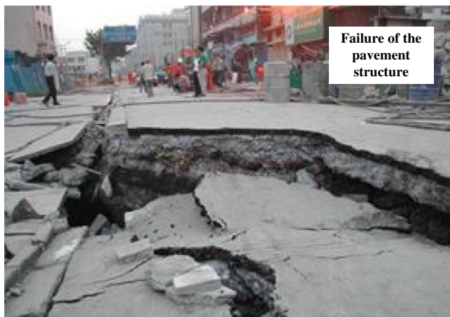
Fig. 22 Damages caused by the collapse of the tunnel of the Shanghai Metro Line 4 (after Xu et al. 2009)
