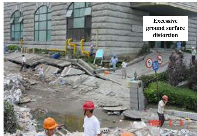
Fig. 22 Damages caused by the collapse of the tunnel of the Shanghai Metro Line 4 (after Xu et al. 2009)
