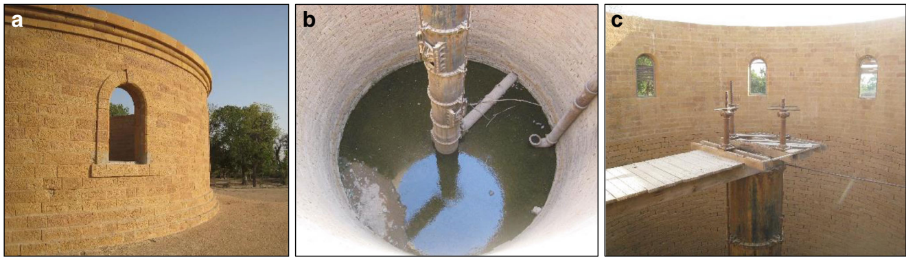
Fig. 6 a–c A view of Dumlottee well (inner and outer view)
