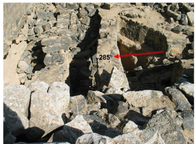
Fig. 5 Arch of underground water reservoir curved in the direction of 285^\circ found excavated in Umm Al-Jimal
