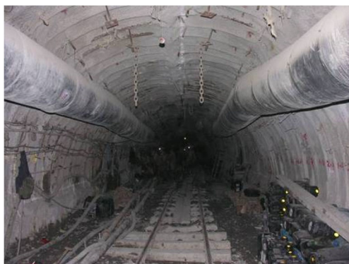
Fig. 25 The completed south haulage underground opening during re-excitation
