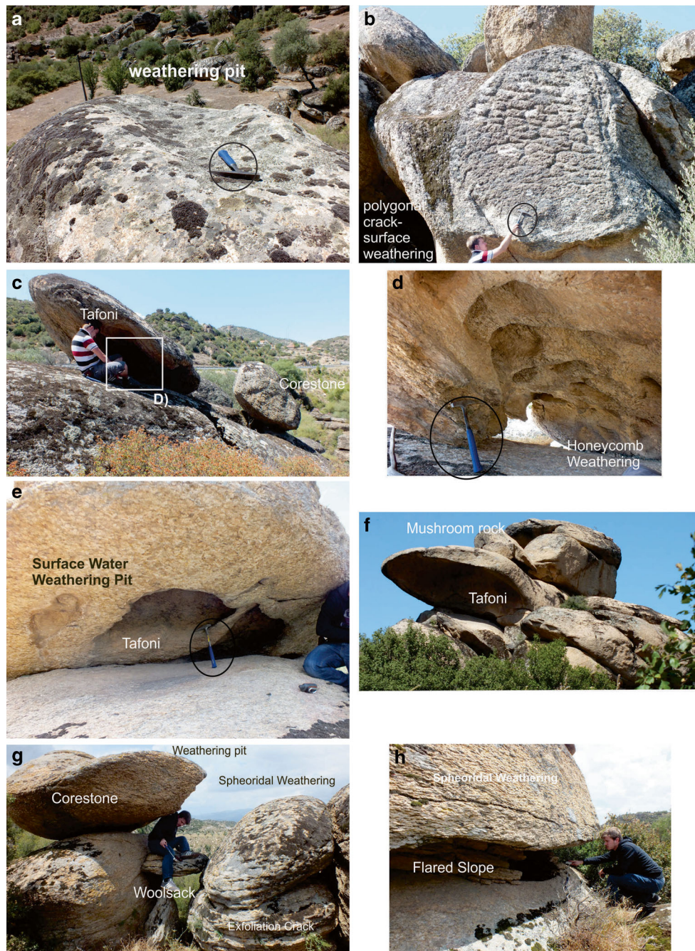
Fig. 6 Field view of the minor geomorphological structures that can be observed both in leucogranites and orthogneiss. a The weathering pit is formed as a result of the surface water flowing and selective erosion with various scales (in orthogneiss, SW Memişler village). The water flowing can create depressions with varying scales (hammer in circle for scale, 33 cm). b The polygonal crack or surface weathering is formed on the surface of boulder block (in orthogneiss, SW Memişler village; hammer in circle for scale, 33 cm). c Some blocks at the top of the rock contain tafoni with honeycomb weathering (in orthogneiss, N Hacıaliler District). d The close inside view of the tafoni includes honeycomb weathering (hammer in circle for scale, 33 cm). e A meter-scaled tafone includes honeycomb weathering and water trace. Two small depressions are observed at the left of the tafoni (in orthogneiss, N Hacıaliler District;
