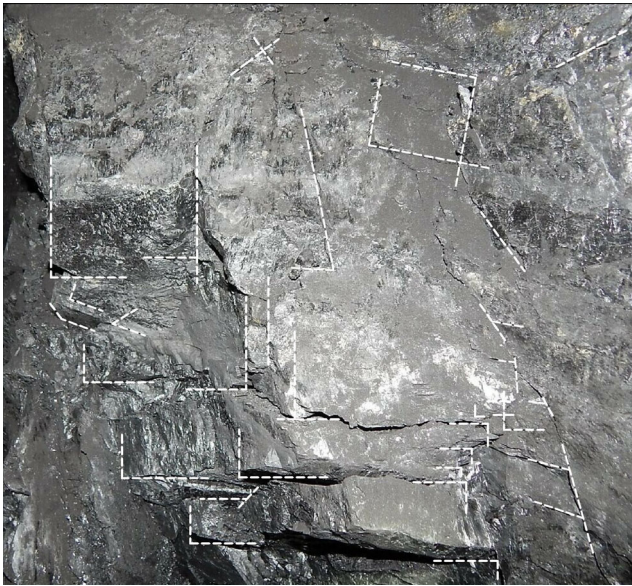
Fig. 1 A photo that mainly contains simplified orthogonal fissures (in the protective coal pillar at tunnel 5937 of Tashan mine in China)
