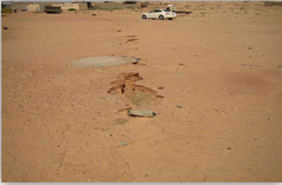
Fig. 1 An overall view of a crack extending more than 45 m
