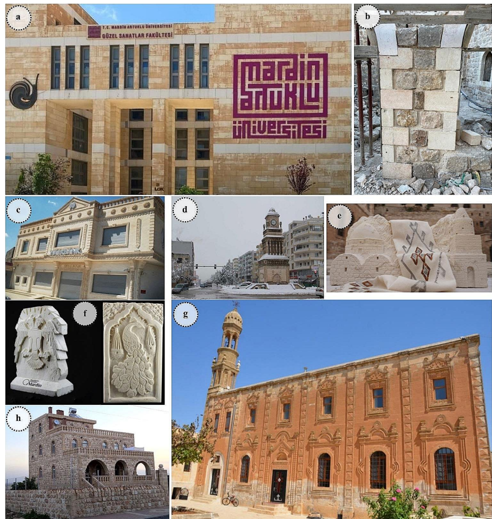
Fig. 9 Contemporary use of the Mardin Stone. (a) The campus of Mardin Artuklu University; (b) The application of the Mardin Stone in the restoration of a historical structure; (c) A bank branch in Midyat; (d) A clock tower at the city center of Midyat; (e-f) Miniatures carved into the Mardin Stone ( http://tinyurl.com/4ujzm6yh ); (g) Mor Şarbel Church, Midyat, the last church built in the study area; (h) A modern masonry structure in a Syriac village constructed with the Mardin Stone
