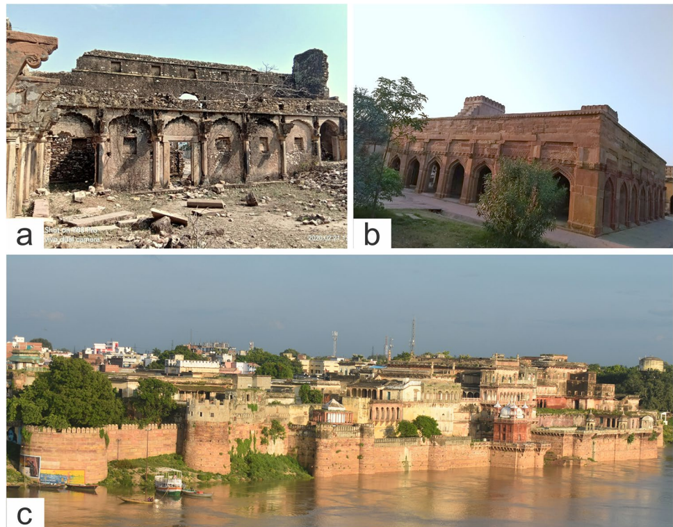
Fig. 10 Historic forts built in Chunar sandstone ( Balua Pathhar ). a Vijaygarh fort, b Chunar fort and c Ramnagar fort
