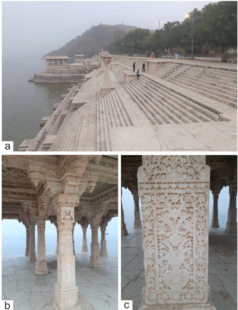
Fig. 9 a Rajnagar marble used in stepped embankment of Rajsamand Lake. b Intricately carved pillars of the pavilion of Nau Chauki . c Close-up view of one of the carved pillars at Nau Chauki (photos by Parminder Kaur)
