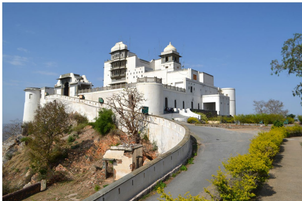
Fig. 12 Sajjangarh Fort with Ghutai -plastered exterior (photo by P.S. Ranawat)
