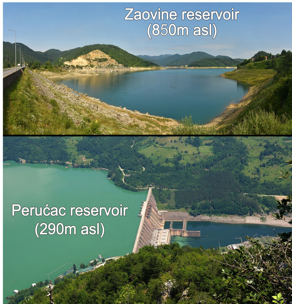
Fig. 9 Reservoirs in the study area. Perućac dam is the main scene of energy production, while Zaovine is a pumped-storage reservoir. Cretaceous sedimentary rocks can be seen in the background mountain of Zaovine. (Photos by Telbisz)
