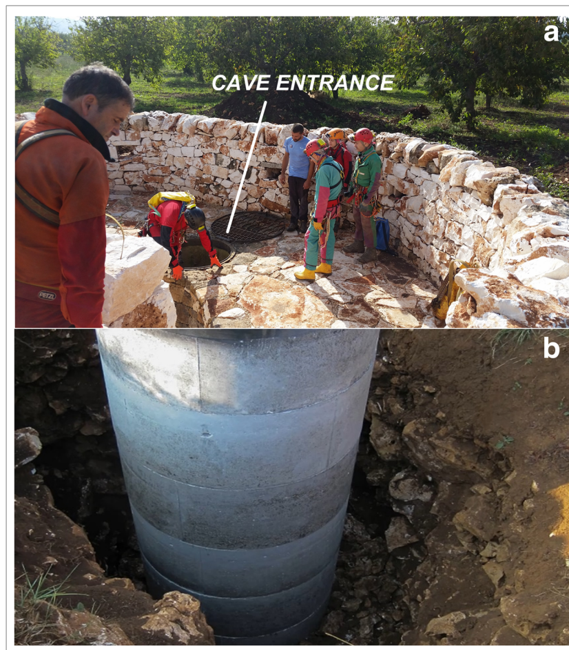
Fig. 2 (A) Dry stone wall surrounding the cave entrance; (B) cement rings located at the entrance of Inghiottitoio di Masseria Rotolo, in order to reinforce it and protect the access of speleologists
