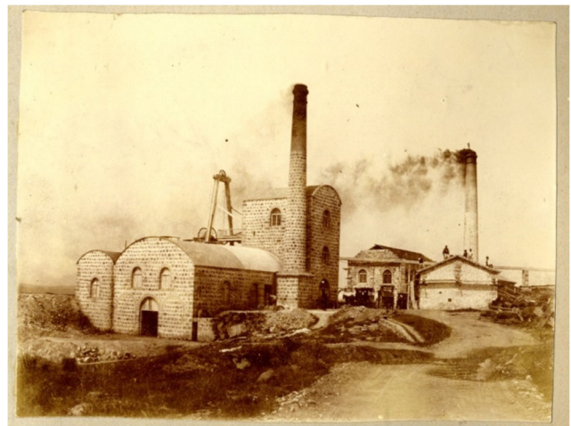
Fig. 13 Engine and boiler houses in La Tortilla mines at the start of twentieth century
