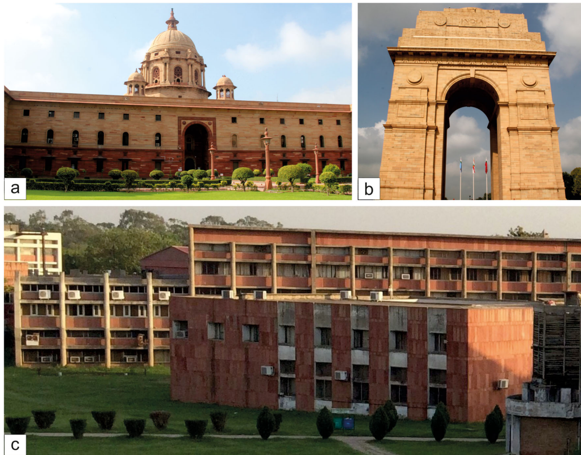
Fig. 10 Photographs showing use of Vindhyan sandstones in contemporary buildings. a Central Secretariat, (b) India Gate in New Delhi, and (c) Panjab University campus, Chandigarh
