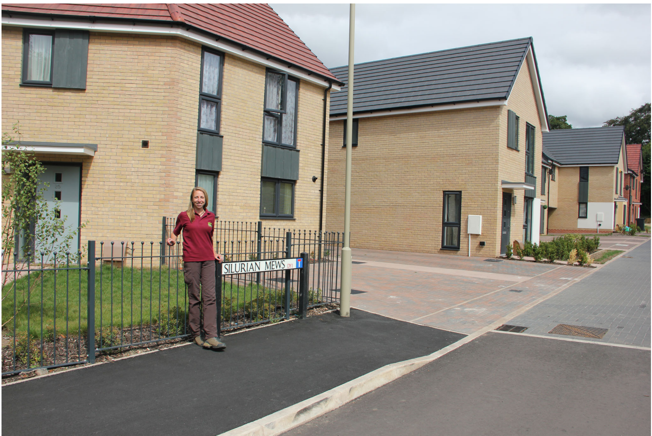
Fig. 6 New housing adjacent to Wren's Nest NNR in the heart of the Black Country UNESCO Global Geopark Project. Here, street names provide the community with connections to the local geoheritage and the quarries that exposed it
