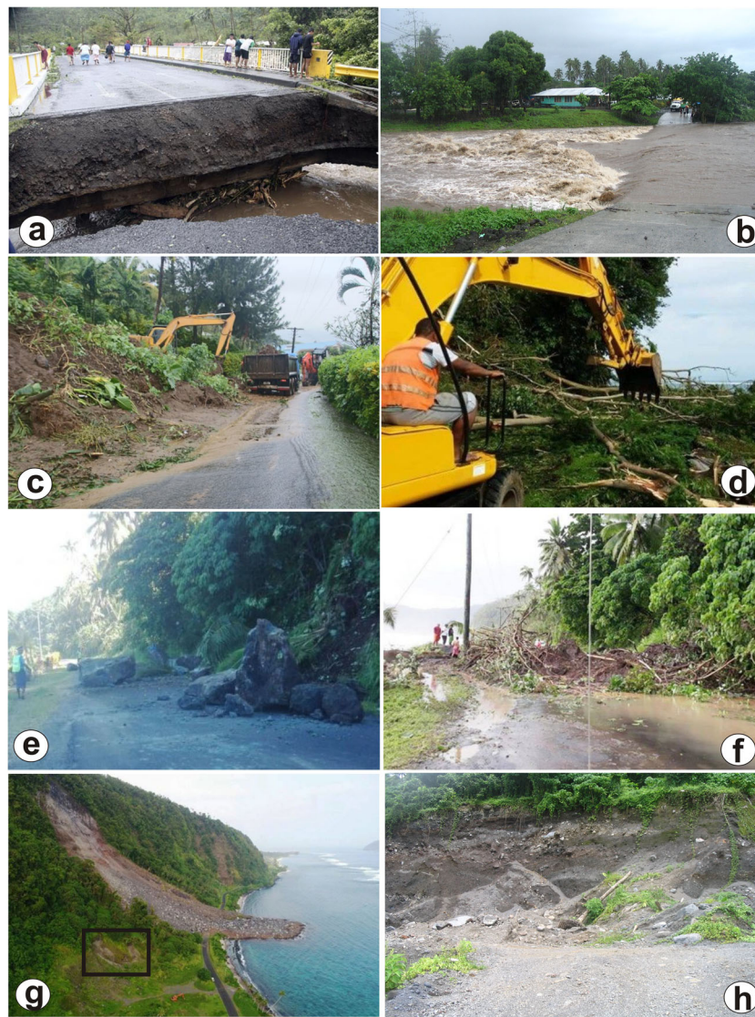
Fig. 2 Wet season in Samoa can generate surface flooding, landslide, and rockfall. a Leone Bridge in the Apia urban area became unstable and disconnected during heavy flooding of Cyclone Evan on the 13th of December 2012 (source: AP Photo/Seti Afoa). b Low concrete bridges and fords are common across Samoa and they are commonly submerged during flood events causing major disruption of transportation such as it happened in 2005 in near Manase, Savai'i (photo: K. Nemeth). c Landslide at the foothill of Mauga-o-Vaea (Mount Vaea) at Palisi area in the southern part of Apia narrowing one of the main road during heavy rain in May 2017 (source: Samoa Observer). d Landslide/rockfall and uprooted of trees on the northern part of Savaii at Manase-Safotu section during Cyclone Amos in April 2016 (source: http://www.talamua.com/samoa-cleans-up-after-a-weakened-cyclone-amos/ ). e Typical rockfall on sealed road in Upolu (Photo: Fefiloi Kerstin from http://www.samoaoobserver.ws/en/04_01_2018/local/28459/Landslide-scare-on-east-coast.htm ). f Landslide at Solosolo at 11th February 2019 disrupted traffic to the east of Samoa (Photo: Land Transport Authority - http://www.samoaoobserver.ws/en/12_02_2018/local/29926/Second-cyclone-reports-dismissed.htm ). g One of the largest landslides occurred near Lalomanu on 12th February 2018 (Source: Land Transport Authority, Samoa). h Volcaniclastic successions exposed along the main highway near Lalomanu in 2005 in a place where recent landslide occurred in 12th February 2018. The bedrock geology is largely unstudied so far (photo: K. Nemeth)
