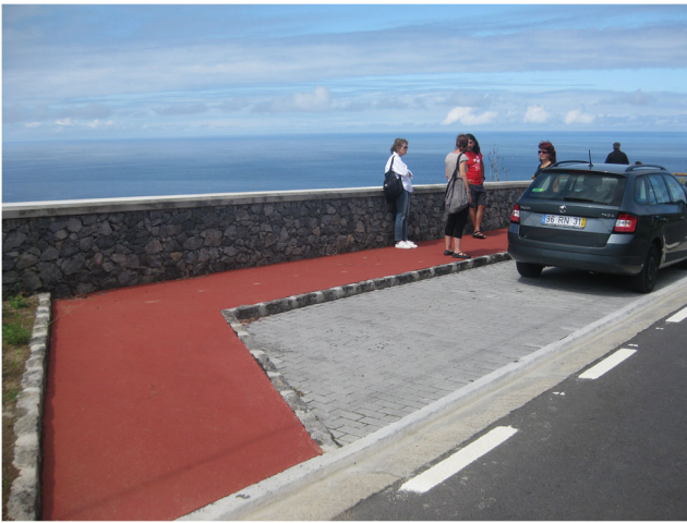
Fig. 5 Facilities provided to people with special needs in a viewpoint located at the Regional Route 1-1 (Azores UNESCO Global Geopark). The installation of ramps in the parking facilitates the access to people with wheelchairs
